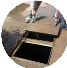
Carefully open cover of the oil separator
